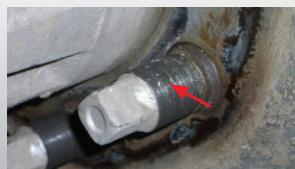
• Rust & Dirt on the Thread
